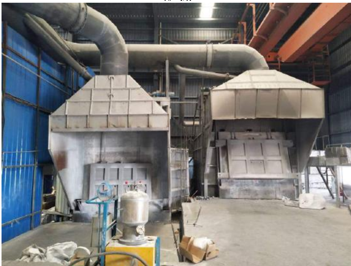
熔炼炉集气罩
